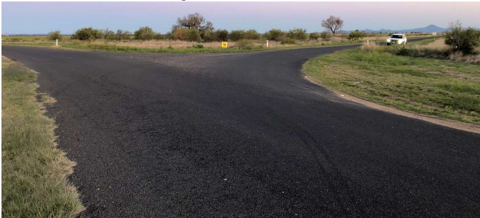
Figure 17: Minor road deformation over culvert at Boo Boo-Gurley Creek road intersection
